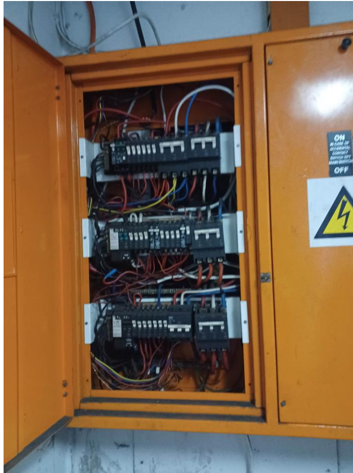
Figure 2: Main DB on the Ground Floors with no cover.
