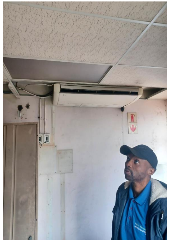
Figure 6: 3 rd floor AC isolator disconnected.
