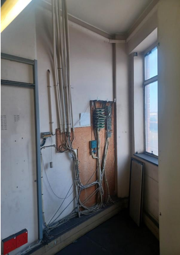
Figure 7: 3 rd Comms Cables Not Housed Properly.
