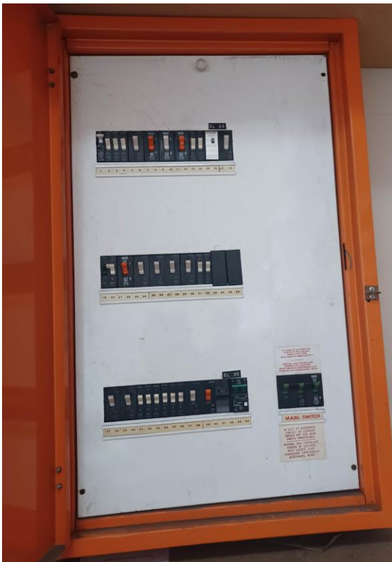
Figure 5: First Floor DB in good condition.
