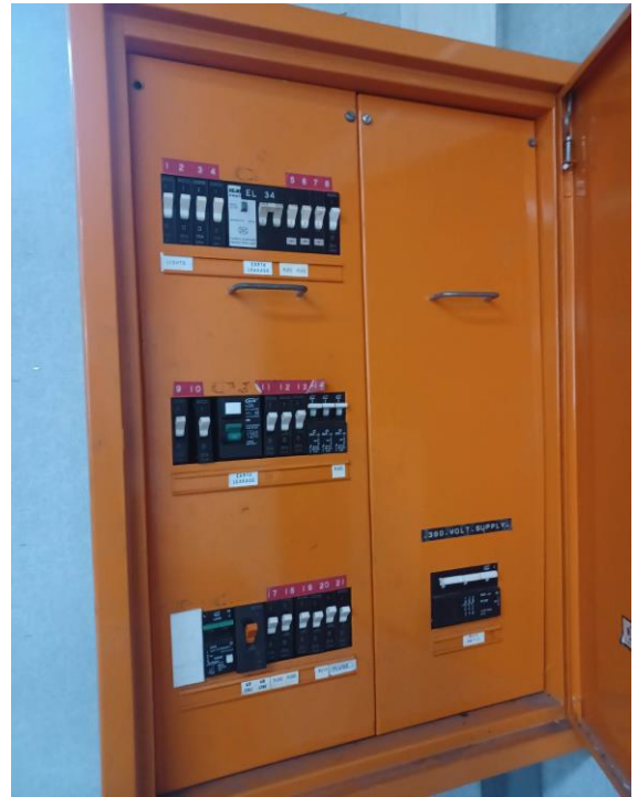
Figure 4: Ground Floor DB in good condition.
