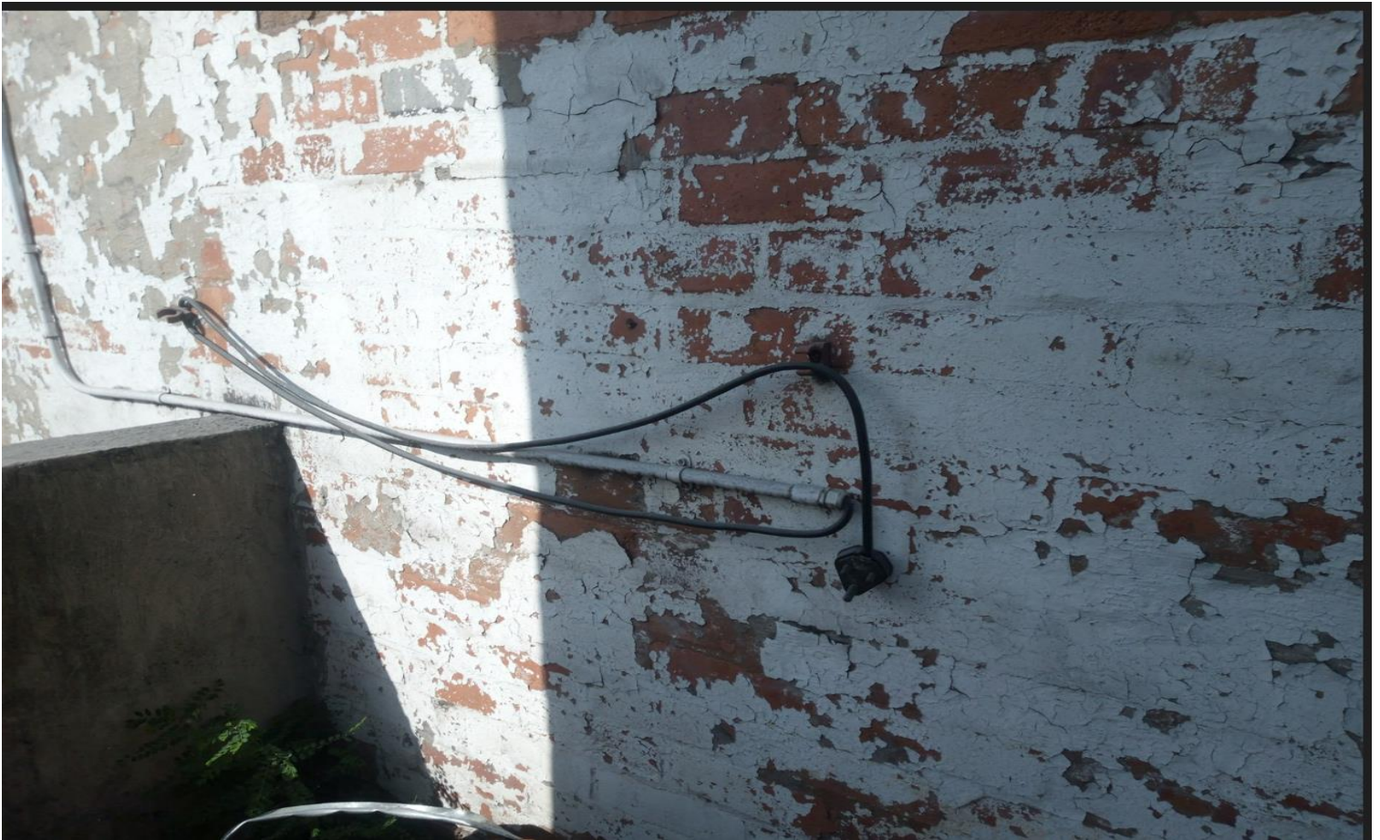
Figure 2: Plug Top where portable generator normally connect to flood lights
